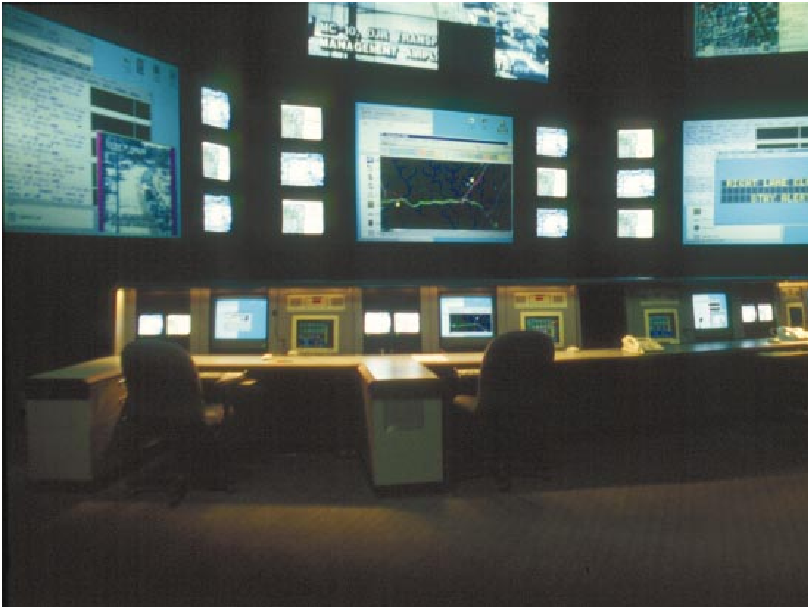
Looking like the bridge of the Starship Enterprise, the State Highway Administration's high-tech Statewide Operations Center allows operators to monitor highway conditions around the clock, seven days a week.
